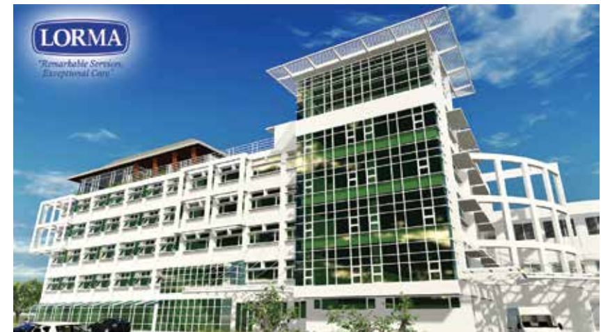
Two-hundred-bed main hospital building
